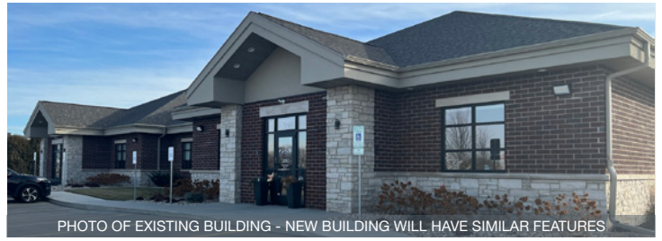
PHOTO OF EXISTING BUILDING - NEW BUILDING WILL HAVE SIMILAR FEATURES
